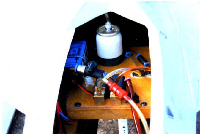
Much of installation pushed right to front
